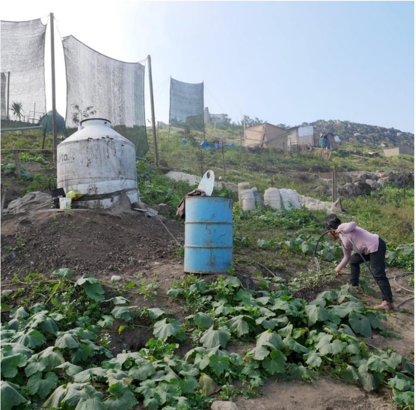
Fog catchers (*atrapanieblas*) are fairly simple constructions. They consist of large plastic or nylon nets stretched between two vertically positioned poles, perpendicular to the direction of the incoming, airborne extension of the ocean,
